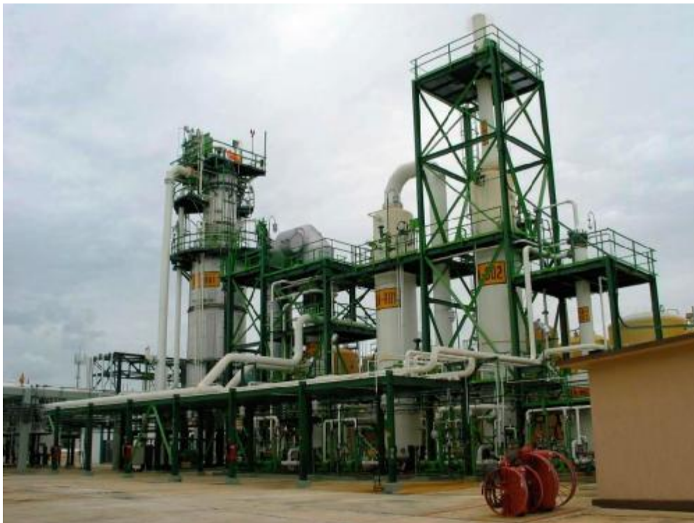
Waste Incinerator III in October 2003.
