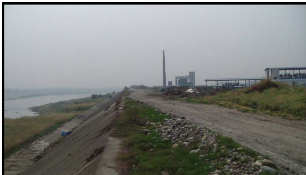
Sichuan Dimeite Biological Science and Technology plant is very close to the Min River (photo by Mao Da)
