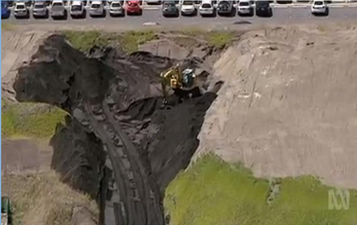
**Open 'dig and dump'.** Has a high potential for mercury releases and impact on human health.
