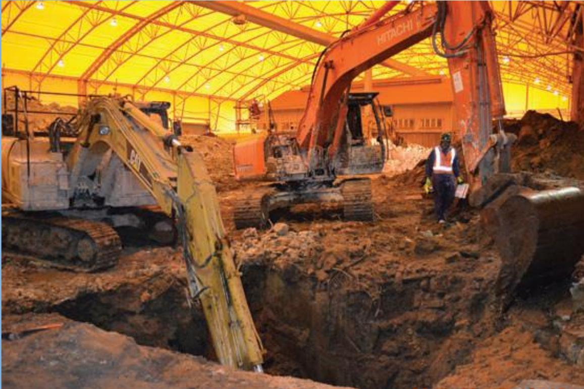
**Best Practice** – Negative pressure remediation enclosure with carbon filters to prevent Hg release impacts on the environment and public.
