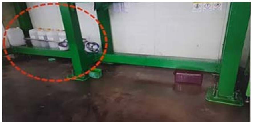
Oil and chemical leaks around production facilities at Samsung's Ho Chi Minh City plant are left unattended.
