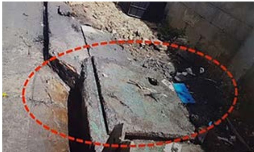
Unattended manholes at a Samsung Electronics supplier are contaminated by spills of pollutants.
