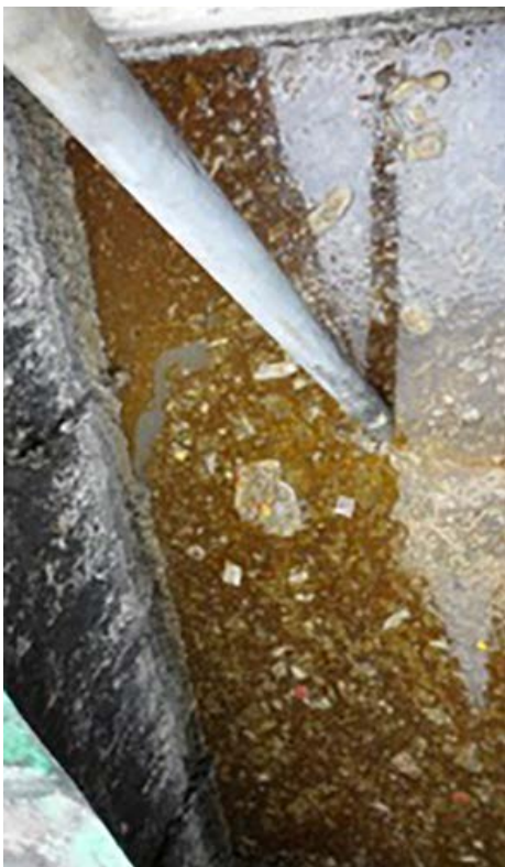
Sewage building up inside tank (left). Overflow of this tank (upper right) with soil contamination (lower right) caused by overflowing sewage tank at the Bac Ninh factory.
