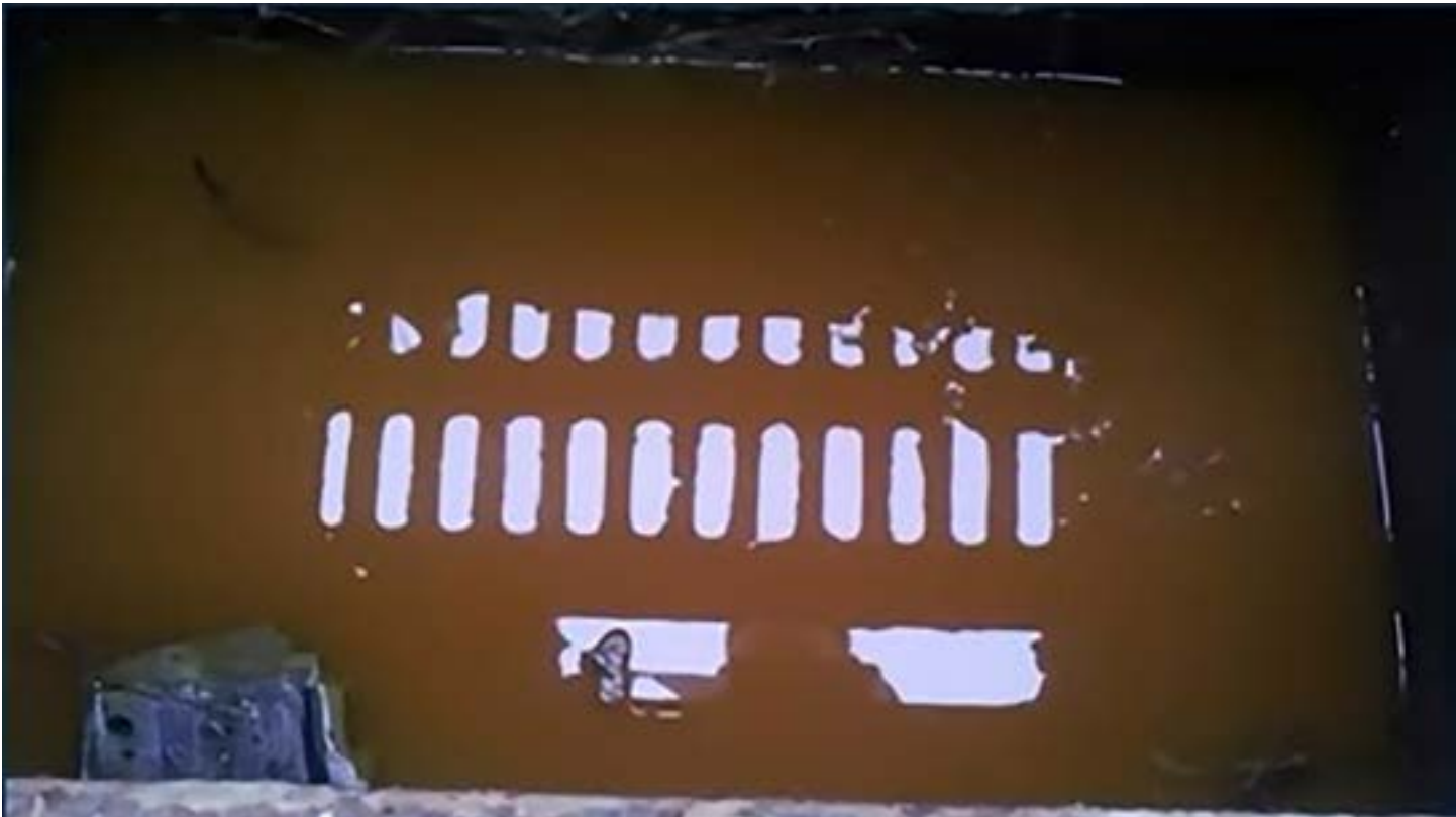
Wastewater leaking from the painting process wastewater treatment facility contaminating the storm drainage system.
