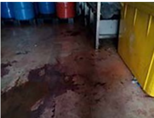
Waste chemicals pooled on top of storage containers and spilled inside and outside the storage area, contaminating the floor and the outside environment at Samsung's Bac Ninh plant.
