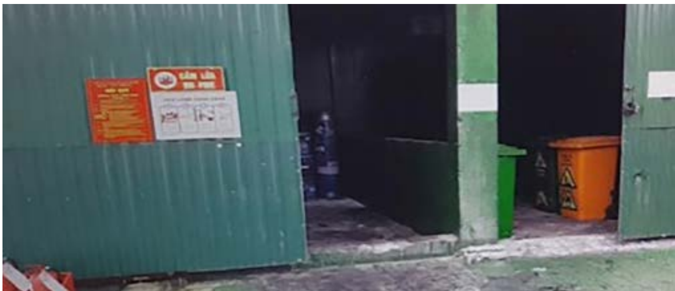
No trench or outflow guard is present to prevent leakage of hazardous substances, allowing pollutants to spread outdoors at a Samsung Electronics supplier.
