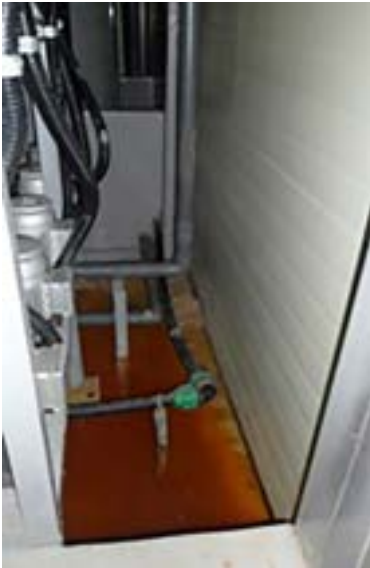
The chemicals to treat wastewater such as NaOH or Al_2(SO_4)_3 leaking from a wastewater treatment facility tank over the leak prevention barrier and out of the facility.
