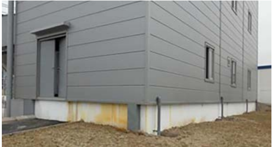
The chemicals to treat wastewater such as NaOH or Al_2(SO_4)_3 leaking from a wastewater treatment facility tank over the leak prevention barrier and out of the facility.
