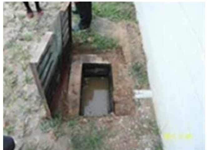
Waste chemical storage (left), a collection tank inside the waste chemical storage (top right), and an external drain connected to a collection tank inside the storage (bottom right).
