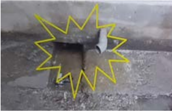
Waste oil and toxic wastewater outlet at a Samsung Electronics supplier goes directly to an outdoor storm drain leading to waterways.
